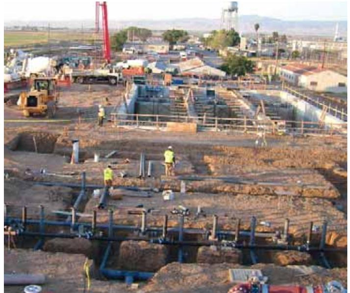
**Underslab piping at membrane building slab with the aeration basin in the background.**
